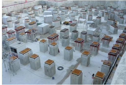
Fig. 3.Columns bear and aseismic pads.
